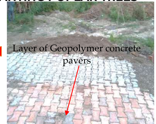
LAYING GEOPOLYMER CONCRETE PAVERS
